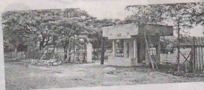
Fachada do campus do IFPR
